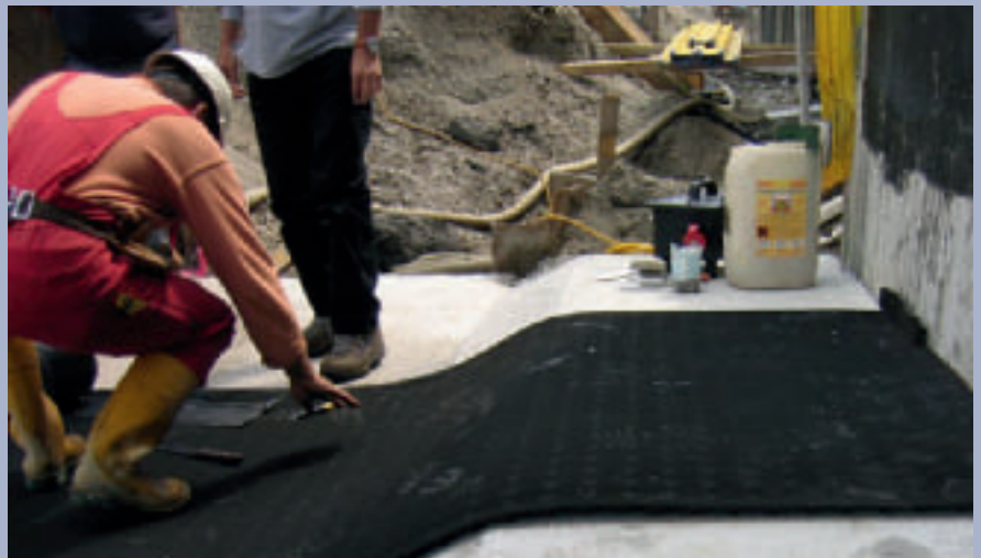
Figure 2: Laying of mats
