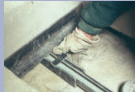
Picture 3: Positioning of the MSS elastomeric Bearings
